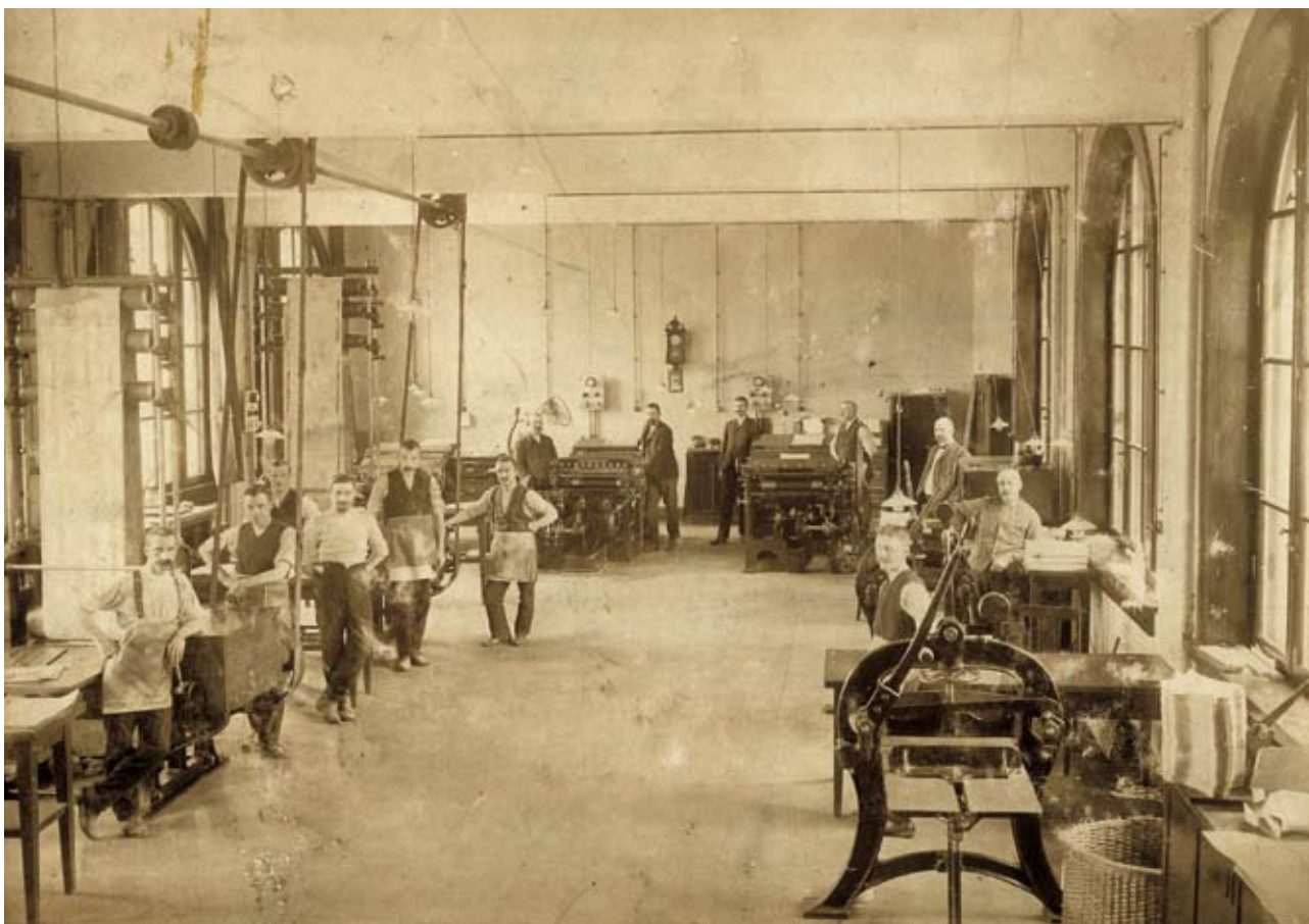
From the new head office at Bankplassen in Oslo when the Printing Works had moved in on the first floor in 1907. Many of the employees from Trondheim moved to Oslo with the Works.
